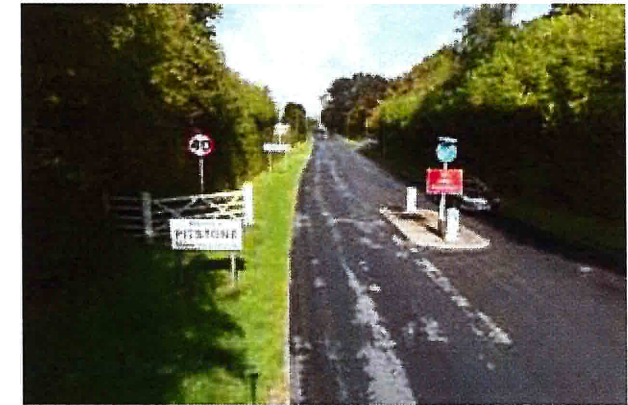
Existing village entrance from west
