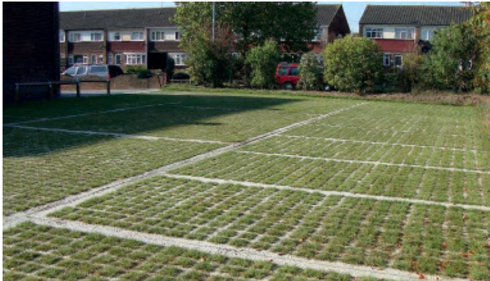
Figure 4-2 Image showing a Grasscrete parking area
