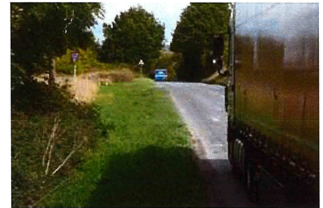
Existing junction difficult to identify
