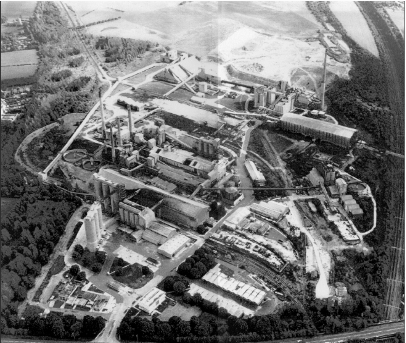
Fig 5. Pitstone cement works
