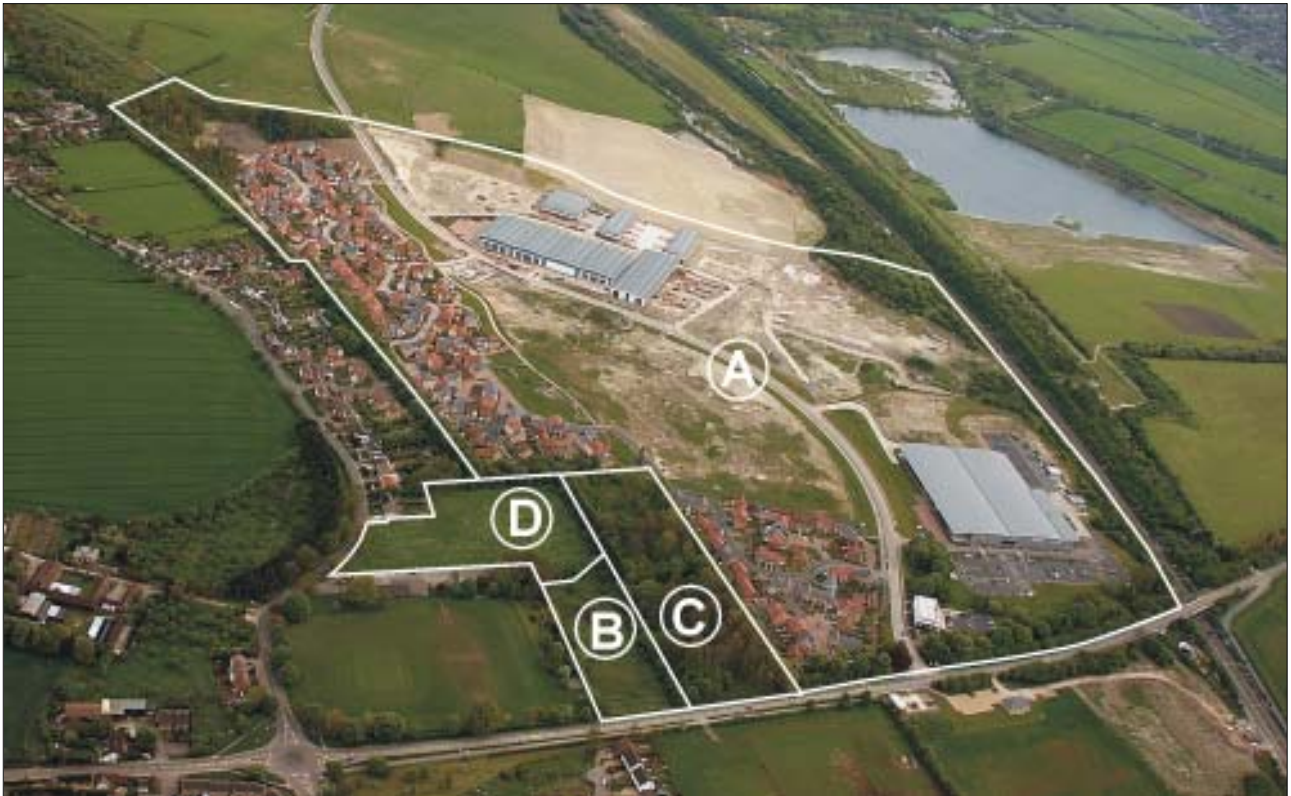
Fig 8. Aerial view of the development area
