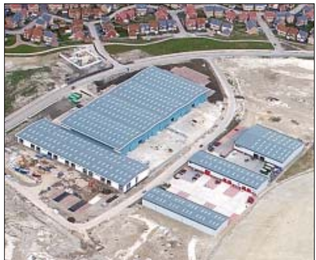
Fig 15. Business development under construction
