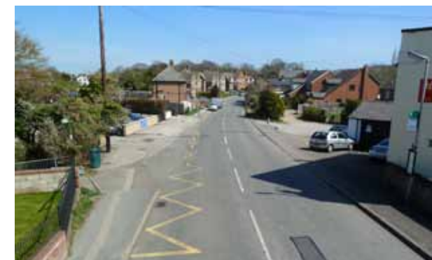
The existing wide and ill-defined space outside the school
