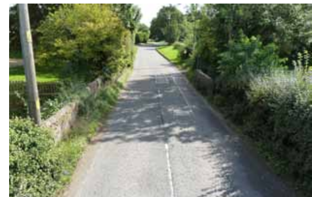
Whistlebrook Bridge- highlight parapets and crossing
