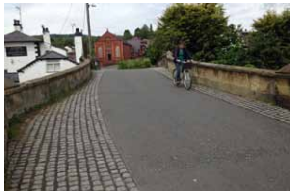
Verge treatment to highlight bridge
