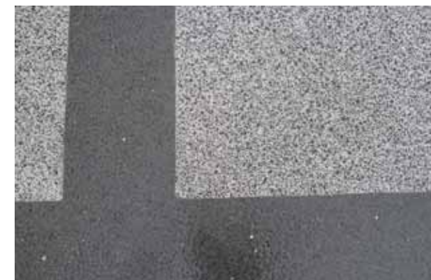
Applied aggregate finishes to existing asphalt
