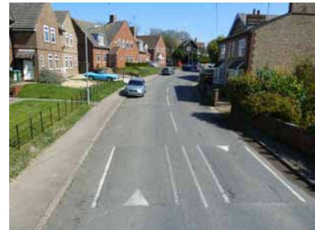
The route up High Street to the centre needs clearer parking and visual narrowing
