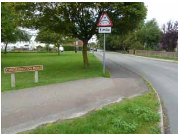
New path along Cheddington Road
