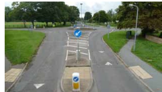
Existing sweeping approach lanes
