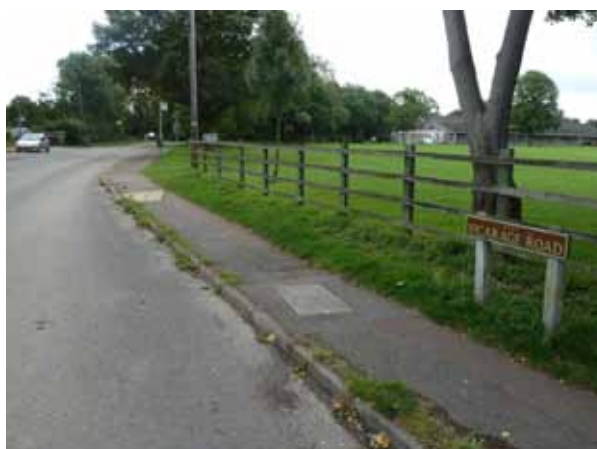
Vicarage Road – Widen footway to 3m. to reach Memorial Hall
