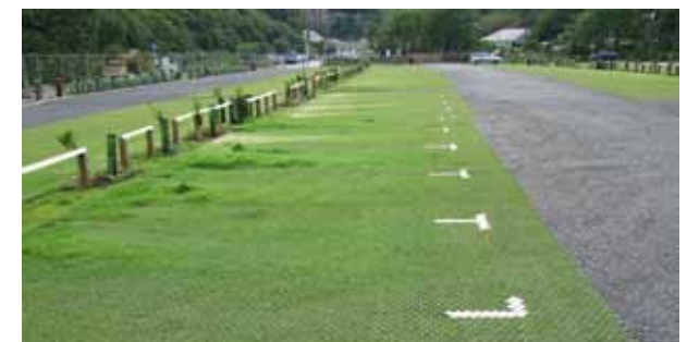
Reinforced grass paving to parking areas
