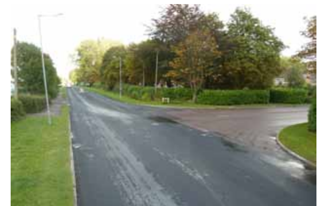
Existing Westfield Road junction
