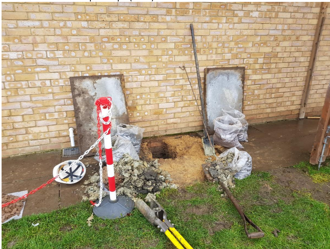
Photo 5: Foundation exposure pit (FDP1)
